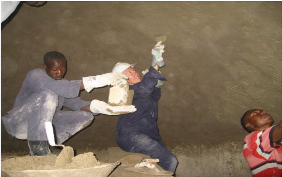
Illustrasjon 5: The tank must be waterproof at the bottom and gas proof at the top. This requires skilled masons to perform proper work.
